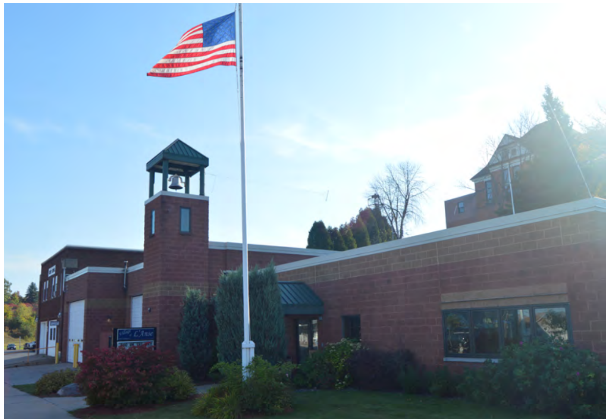
FIGURE 5.3 - VILLAGE HALL & FIRE STATION
