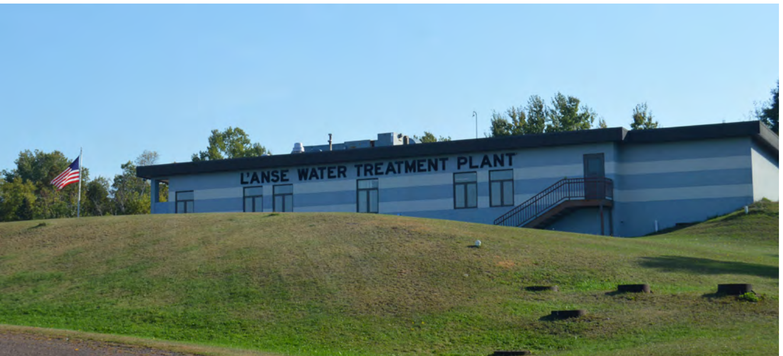
FIGURE 5.0 L'ANSE WATER TREATMENT PLANT
